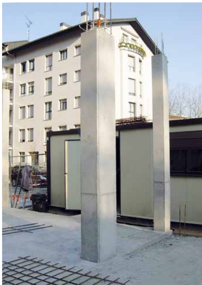
▲ Column finishing with chamfered corners
